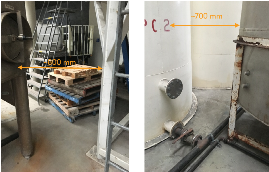
Figure 11-3: Reduced Clear Width of Path of Travel Between Vat 45 & Vat 46 (Left) and Vat 42 & Vat 48 (Right)
