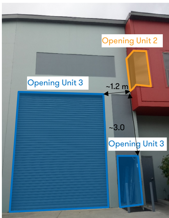
Figure 11-1: Location of unprotected openings.
